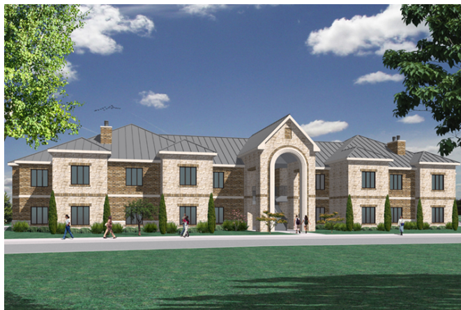
Student Housing Phase II at U. T. Permian Basin
