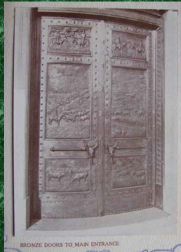
BRONZE DOORS TO MAIN ENTRANCE
