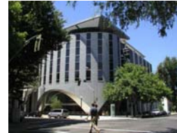
Capital Area East End Complex, Sacramento, CA
