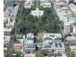
Capital Area East End Complex, Sacramento, CA
