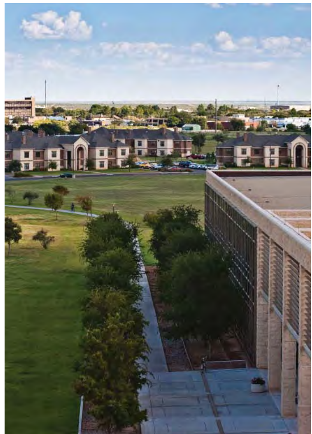
UTPB apartment style housing has been located within easy walking distance of the academic core.
