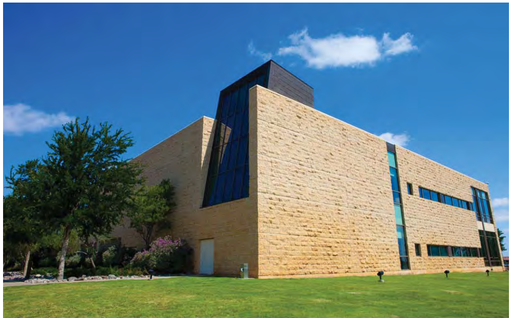
The UTPB Library Lecture Center features a native limestone veneer and copper roof elements.
