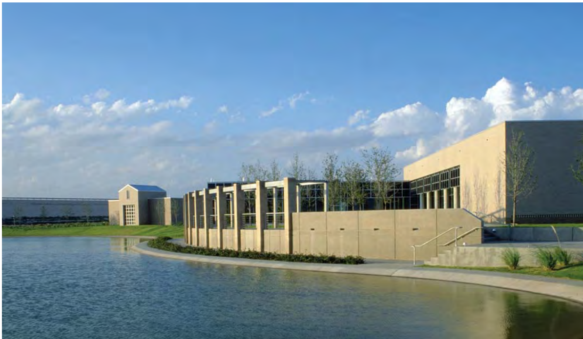
The UTPB Center for Energy and Economic Diversification, (CEED).
