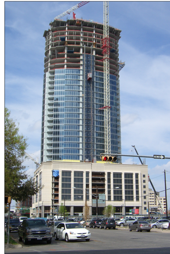
The Austonian is under construction.
