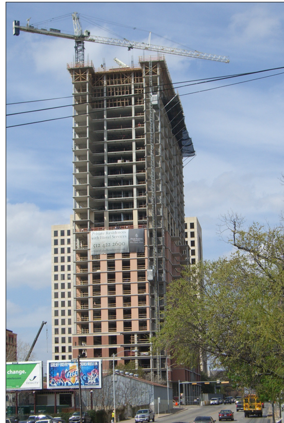
Four Season Residences are under construction.
