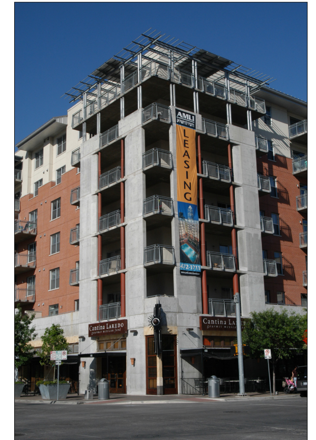
Construction of AMLI on 2nd Street was completed in 2008.
