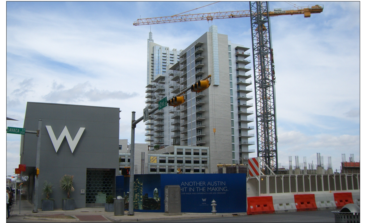
W Austin Hotel and Residences are under construction.
