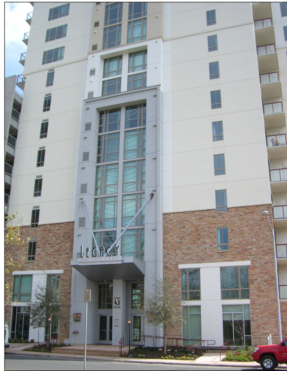
The construction of Legacy on the Lake ended in 2008.
